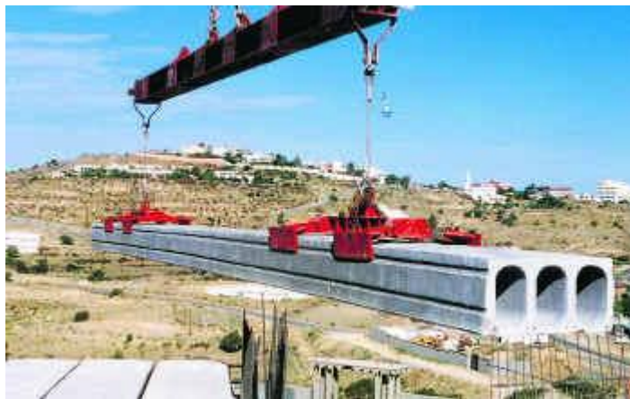
EFFICIENT: Hollow core concrete slabs being used in a building
